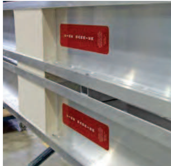
Two hour fire barrier
